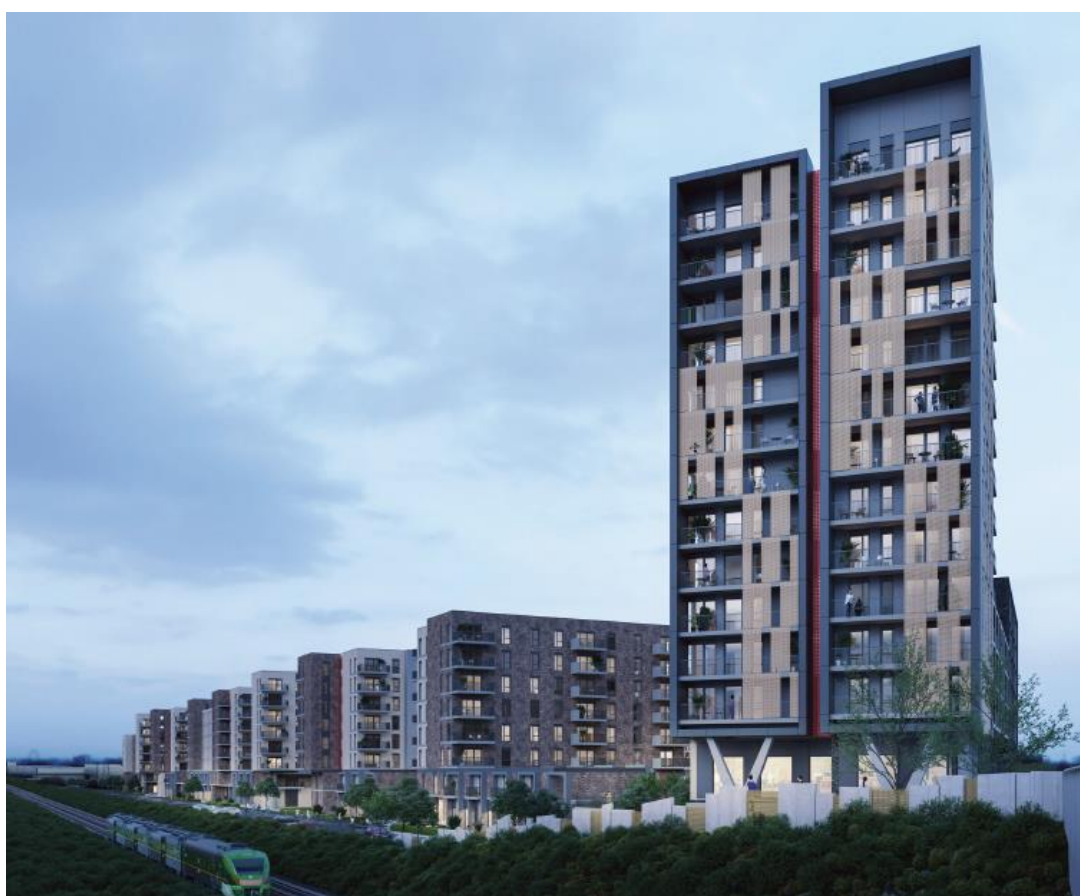
Figure 14.31: Contextual View of North-West Corner of Proposed Development
