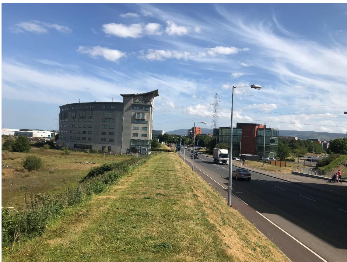
Photo 2: View of the Western Boundary of the Site with Park West Avenue & Aspect Hotel
